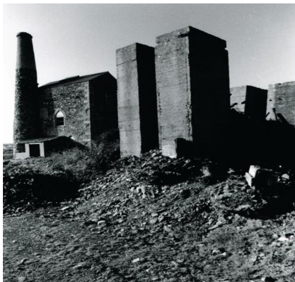
The engine house and crusher supports, Polberro Consols, St Agnes. Image reproduced courtesy of Simon Jones, Cornish Mine Images ( www.cornishmineimages.co.uk )
