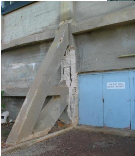
Left: Fire Door Exit for eastern section adapted for the gymnasium. Note the steel reinforcing rods and exfoliated concrete on adjacent buttress.
