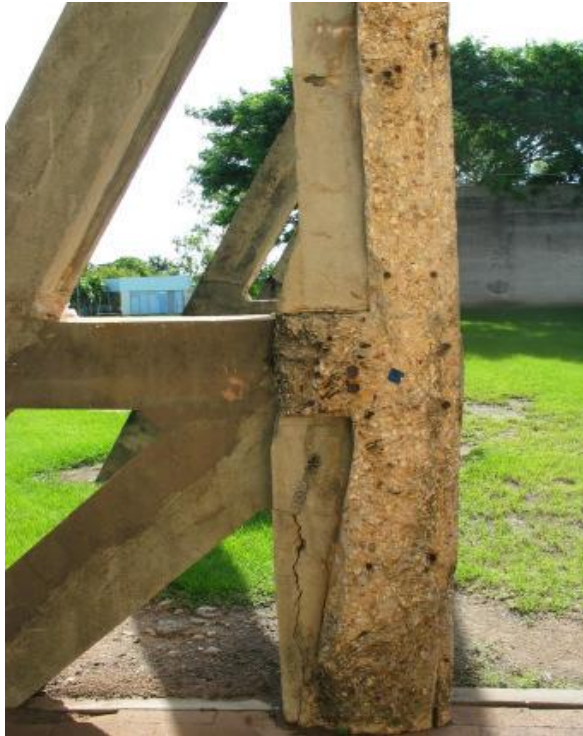
Profile of the concrete wall showing steel reinforcing visible in the open air portion of the Tank (western section) where sections of the south and north wall have been removed.
