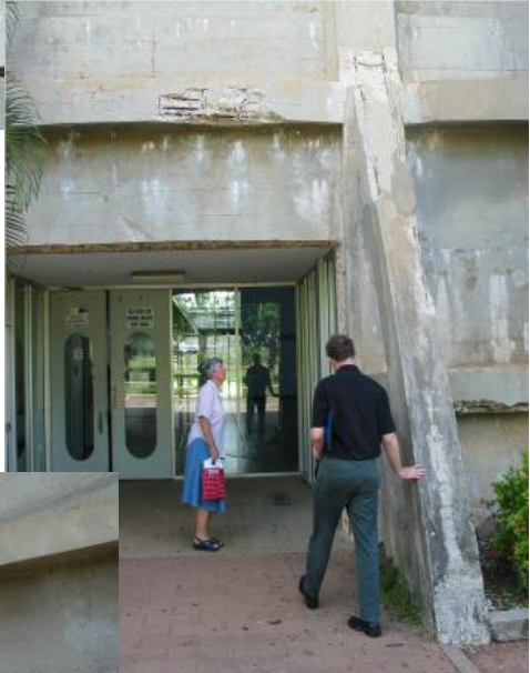
Right: Entrance into the gymnasium section of the Tank. Note the steel reinforcing rods and exfoliated concrete above entrance.
